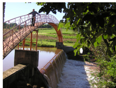
Dam and bridge at Usina Granja Velha.
