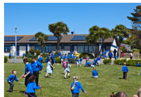
St Columb Minor School benefits from solar PV and a small wind turbine to generate electricity.
