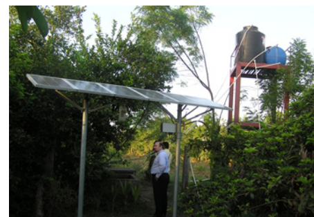
Solar-powered water pump in Chinantlan.
